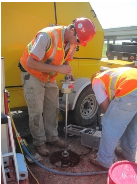
Figure 7. Light weight deflectometer test
