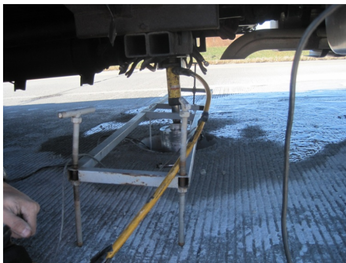
Figure 9. Plate load test
